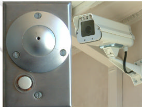
Above: A doorbell/camera and security camera can be viewed on any television throughout the residence.
